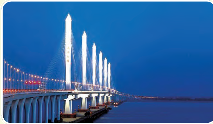
COSCO Kansai Companies Supplying Anti-Corrosion Coatings to the steel structure of Jiaxing-Shaoxing Sea Bridge.
