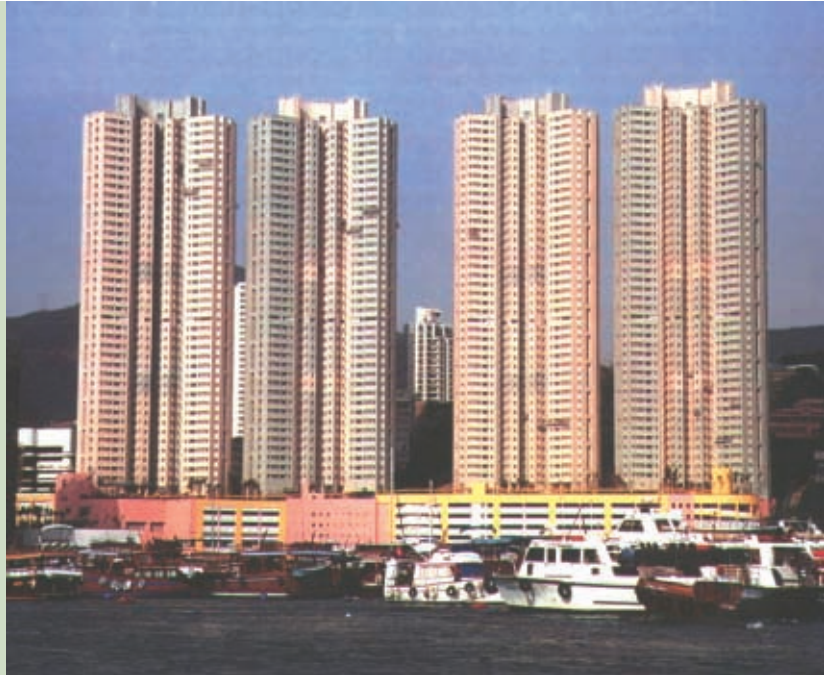
PSPS Project at Shum Wan Road, Hong Kong – Broadview Court
