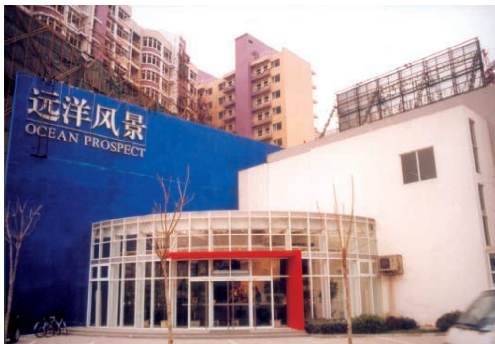
Ocean Prospect, a real estate development project in Beijing
